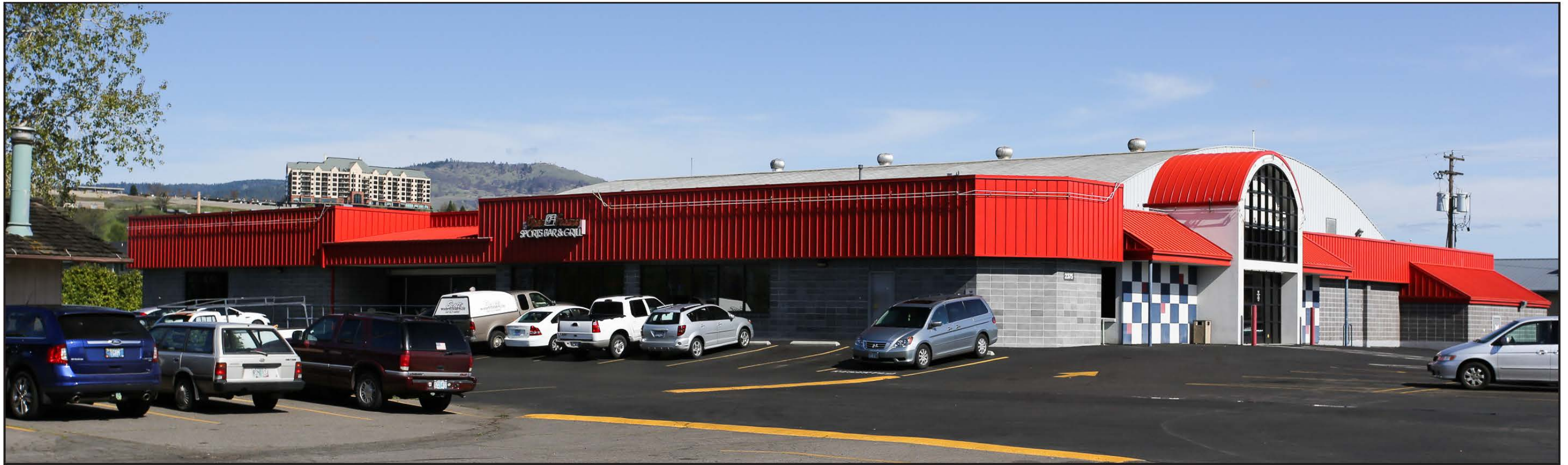
Existing Bowling Alley
